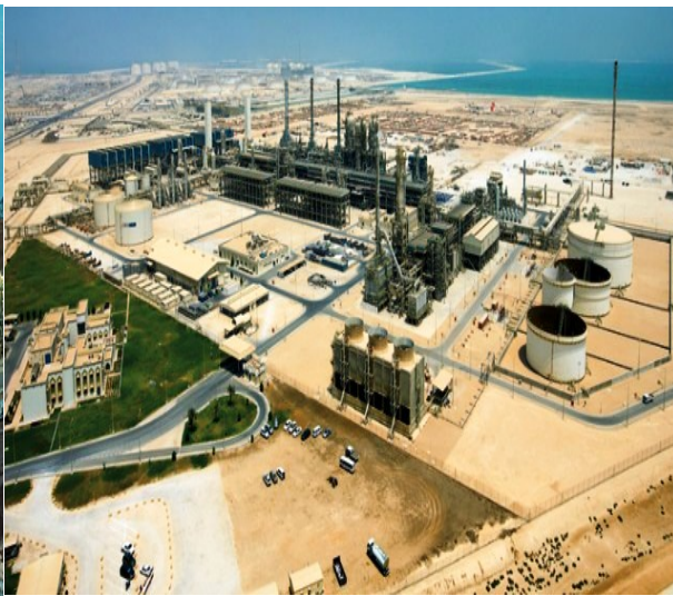
Sasol Qatar 35,000 BPD Gas to Liquids (GTL)
