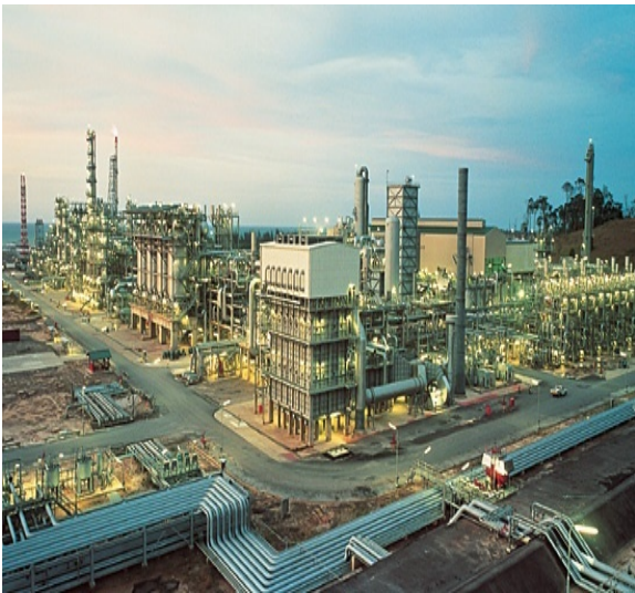
Shell Bintulu 15,000 BPD Gas to Liquids (GTL)
