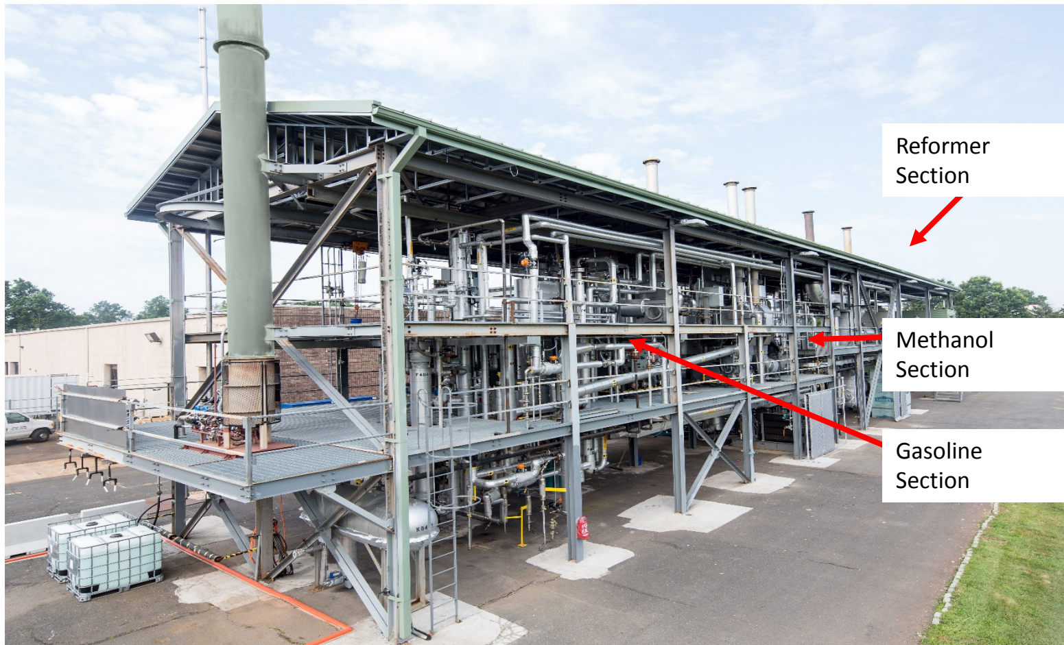
Primus 1,250 bbl/d full scale commercial plant in NJ used as a training center for new operators and for testing new catalysts
